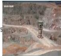
Takaraf's Relocatable Crushing Plant at Cliffe Hill Quarry, UK
