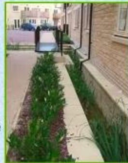
SuDS scheme at Stamford Robert Bray Associates
